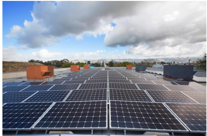
Mitsubishi Electric solar modules cover Chua Di Lac Buddhist Temple & Unified Event Center. The 49.8 kW installation is in San Jose, Calif.
