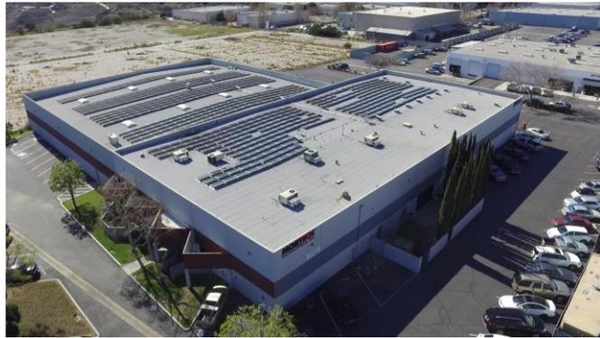
Mitsubishi Electric solar modules cover Mortech Manufacturing's facility. The 183.4 kW installation is in Azusa, Calif.
